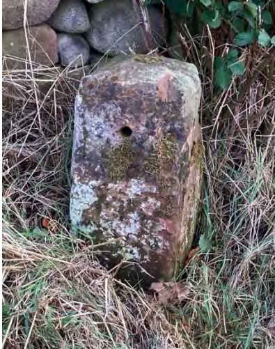
CU_PRCL 08 Boggle Hall layby
